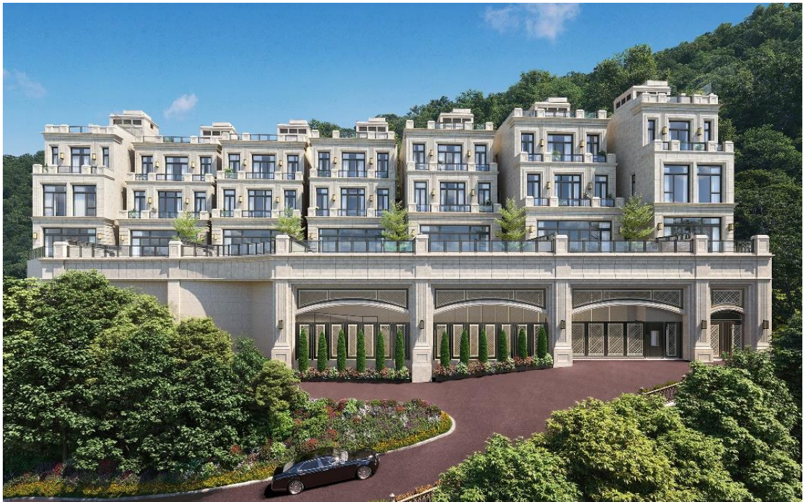
A rendering of MOUNT POKFULAM, a unique luxury house development at Pok Fu Lam Road 1
